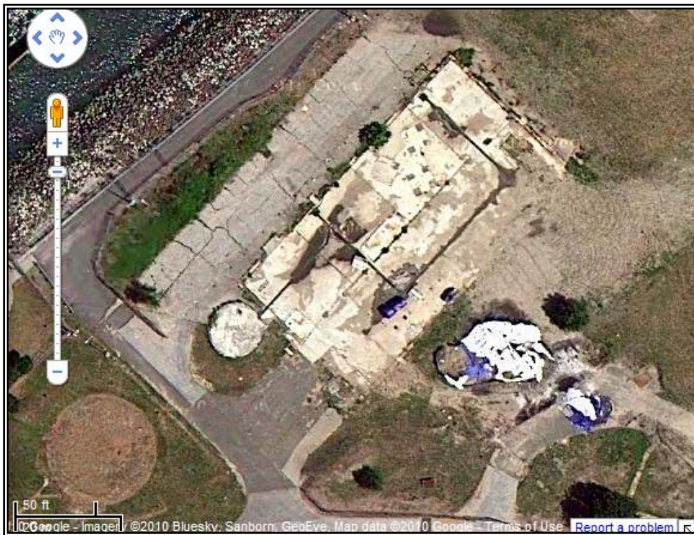
Bottom: Aerial image of Astoria Powerhouse from Google Maps, accessed 2010.
