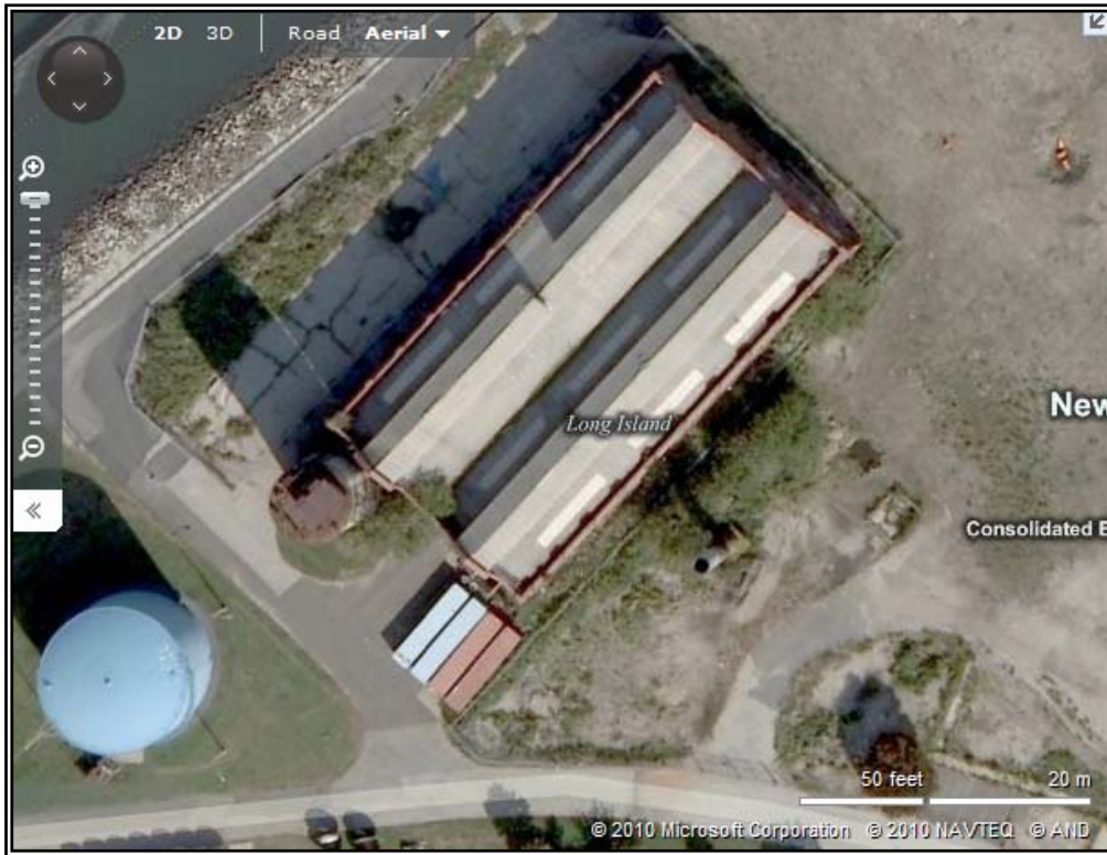
Top: Aerial image of Astoria Powerhouse from Bing Maps, accessed 2010.
